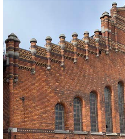
View of facade detailing of building facing the square.
